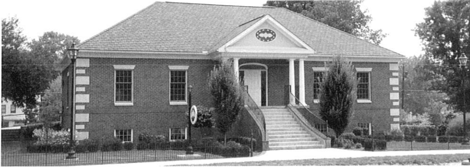
The Muskingum County Community Foundation (Photo by Stephanie Kline)
