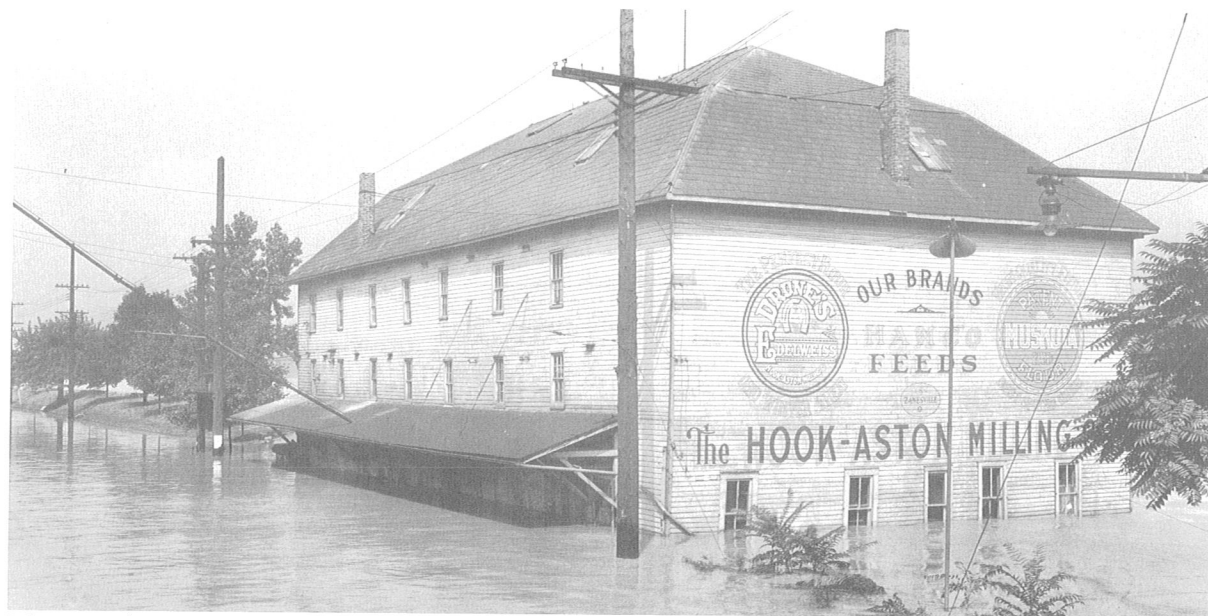
The Hook-Aston Milling Company Building during the Flood, 1935 (located on the west side of the Muskingum River, north of the Baltimore & Ohio Railroad Bridge), Times Recorder
