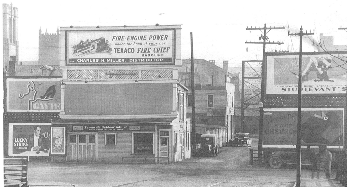
Facing Fifth Street Bridge on State Route 77, Times Recorder
